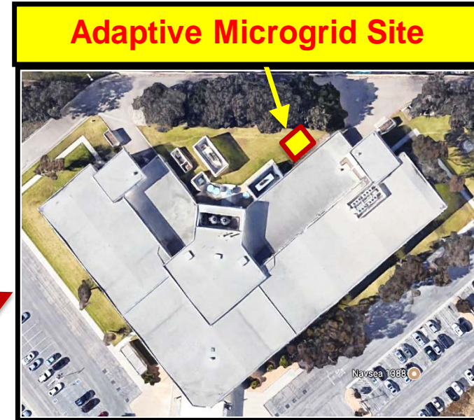
Server Farm Site Location Where EPRI's Adaptive Microgrid With Adaptive Protection Relays, Battery Storage, And Synchronous Condenser Is Planned To Be Installed (Source: EPRI and Google Map)
