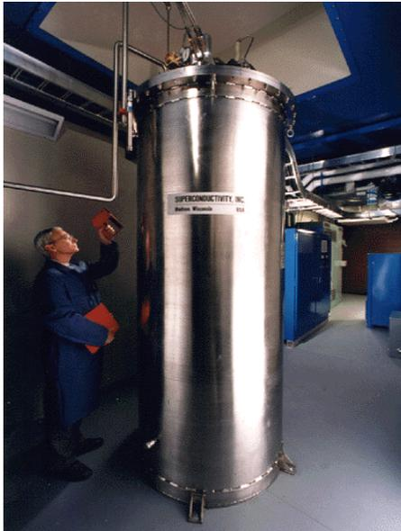
**Figure 3-9: Cryostat holding energy storage magnet in a Distribution Super-Conducting Magnetic Energy Storage System (D-SMES)**
