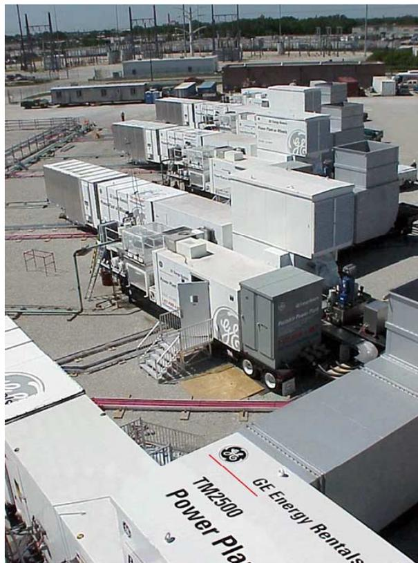
Figure 3-1: Mobile 16 MW gas turbine generators.
