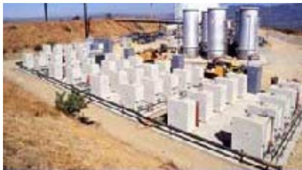
**Figure 2-1: Landfill gas is used to fuel the fifty 30 kW microturbines in this Los Angeles area facility**
