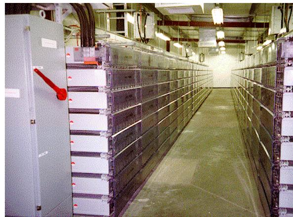
Figure 3-8: VRLA battery bank in a large battery energy storage system (BESS)
