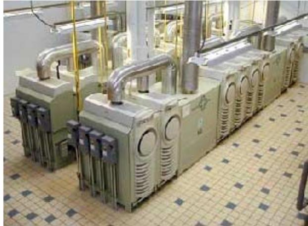
**Figure 2-2: Heat exchangers between groups of microturbines extract exhaust heat which is used to drive a 200 ton absorption chiller.**
