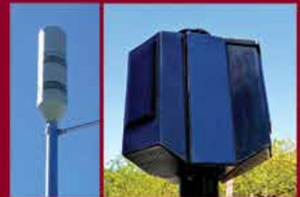
Pole Top Concealment Shrouds Cylindrical and multi-facing 4G/5G Small Cell Concealment Shrouds offer aesthetic housing and rapid deployment of multiple remote radio heads (RRH). Many color options are available to match all types of wooden and metallic poles.
