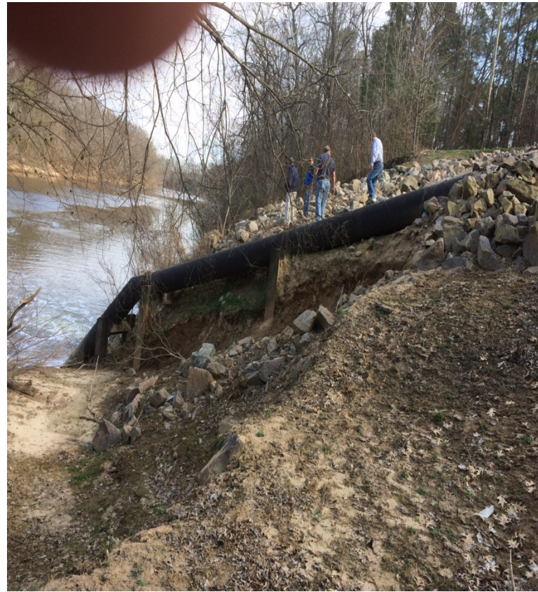
Erosion caused this pipe to become exposed and unsecured
