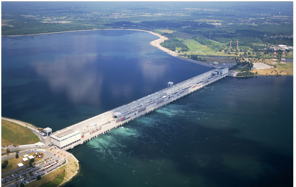
The Moses-Saunders Power Dam, seen from the Canadian side of the St. Lawrence River, which provides power to the St. Lawrence-Franklin D. Roosevelt Power Project. Photo: NYPA https://en.wikipedia.org/wiki/Moses-Saunders_Power_Dam
