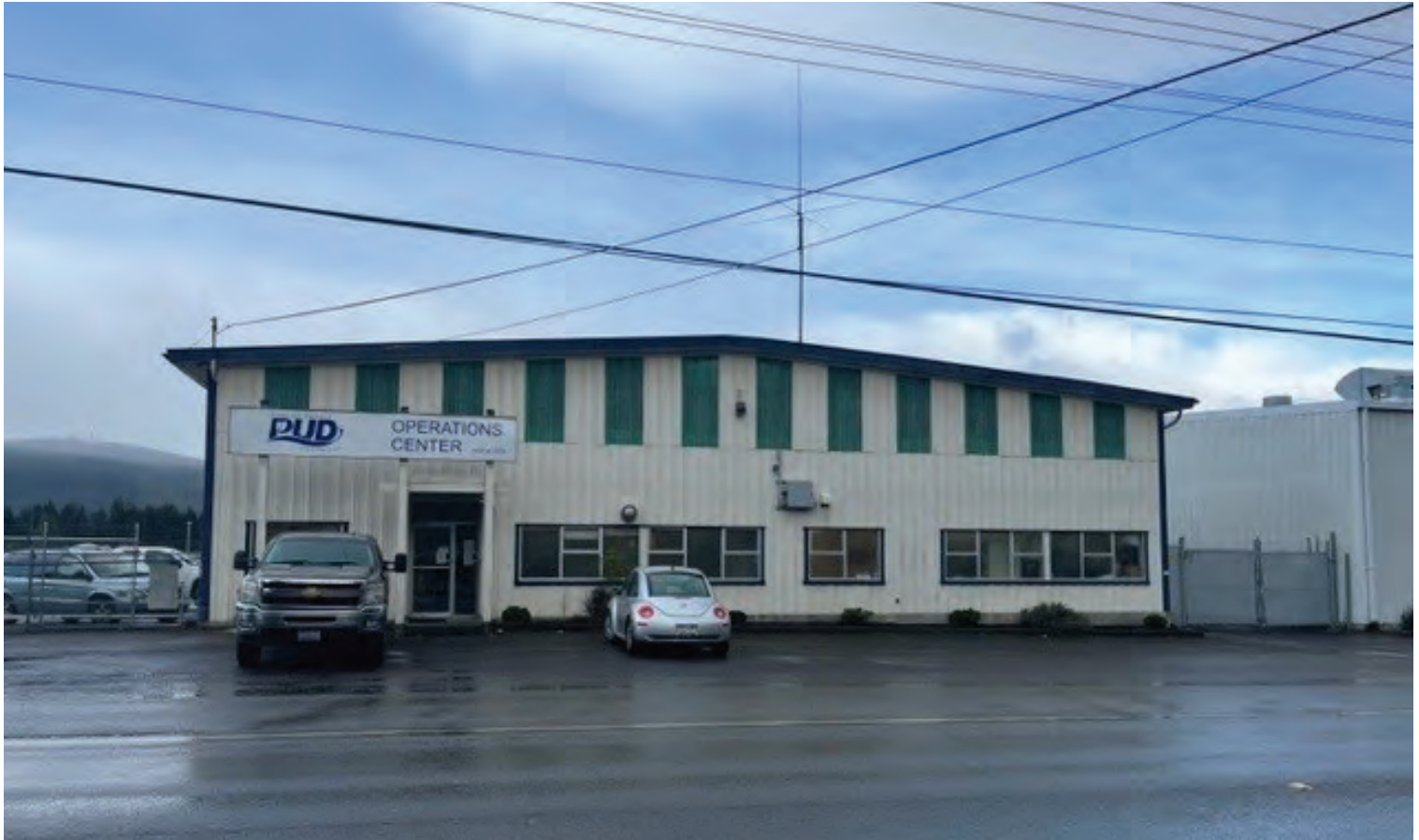
Clallam PUD's original operations center. Photo courtesy Clallam PUD.
