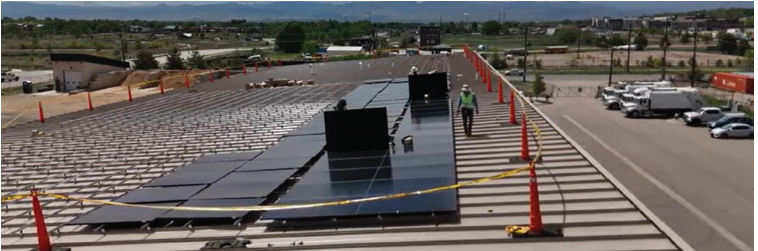
The Longmont, CO Illuminar community solar program under construction. Photo courtesy City of Longmont.
