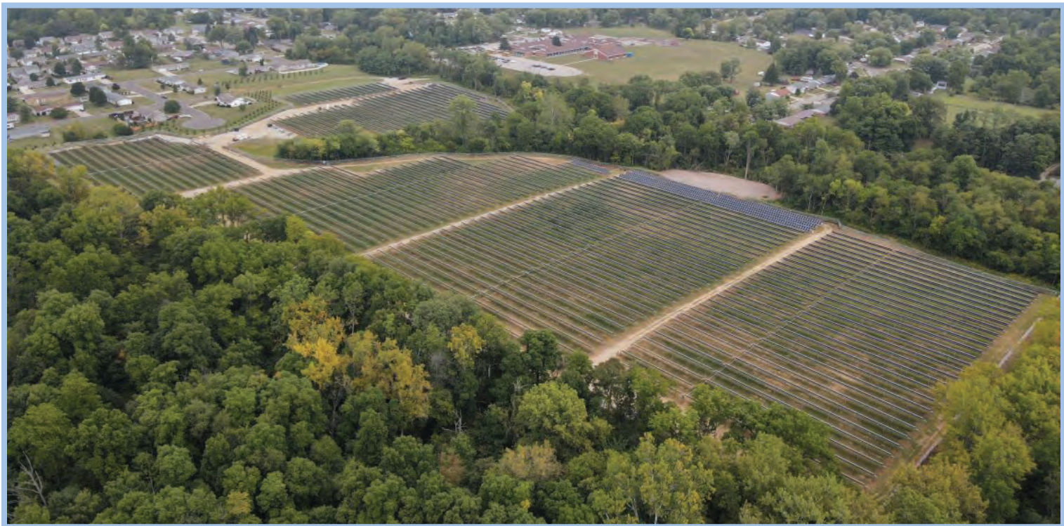
The Richmond Solar Park. Photo courtesy Indiana Municipal Power Agency.
