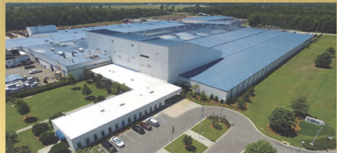
Oranburg, SC Manufacturing Facility
