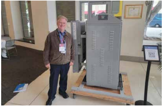
Pasadena Water and Power developed a method to deploy a controllable distribution battery storage system on existing infrastructure.
