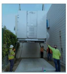
G-417 High Efficiency Recycled Water Indirect Evaporative Cooling System
