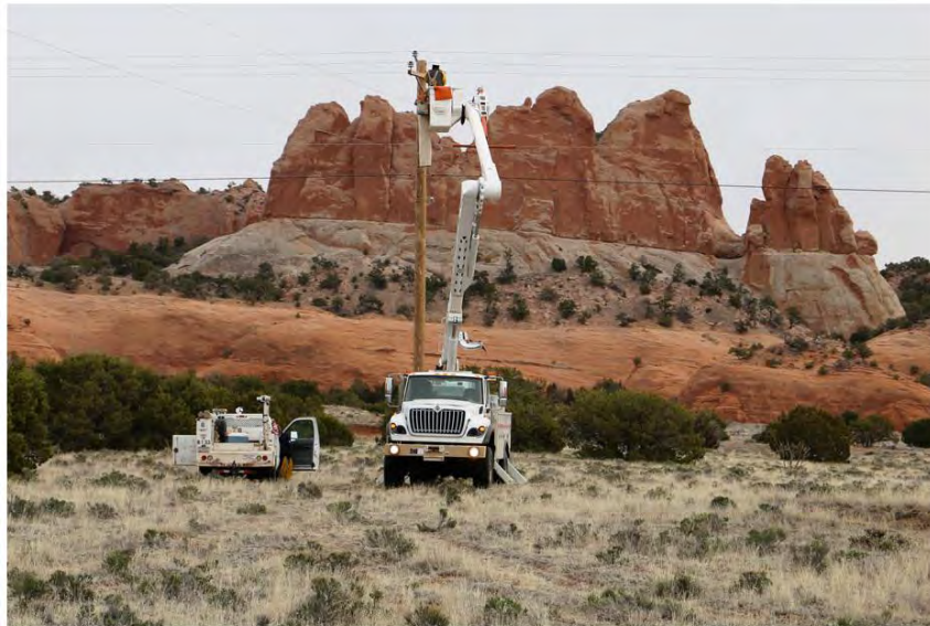
Photo: Alysa Landry/American Public Power Association Workers from Massachusetts connect a distribution line in the Shiprock region.
