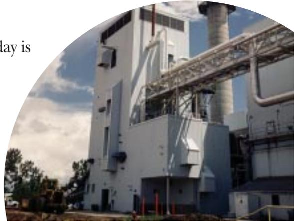
Burlington Electric Department in Vermont has been an industry leader in biomass gasification technology. The utility's McNeil Generating Station can convert wood chips, sawdust, switch grass and other biomass materials into gas for power generation.
