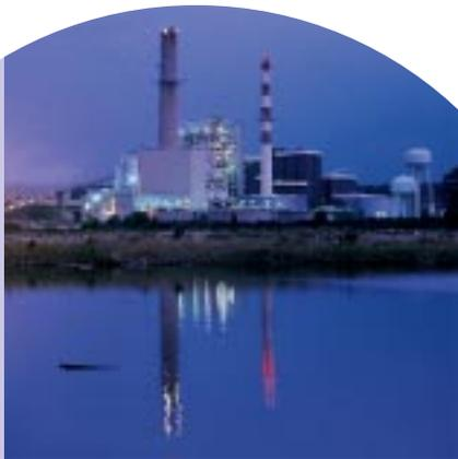
The Deerhaven Generating Station, owned by Gainesville Regional Utilities in Florida, is equipped with controls to prevent formation of nitrogen oxide when burning natural gas or oil.
