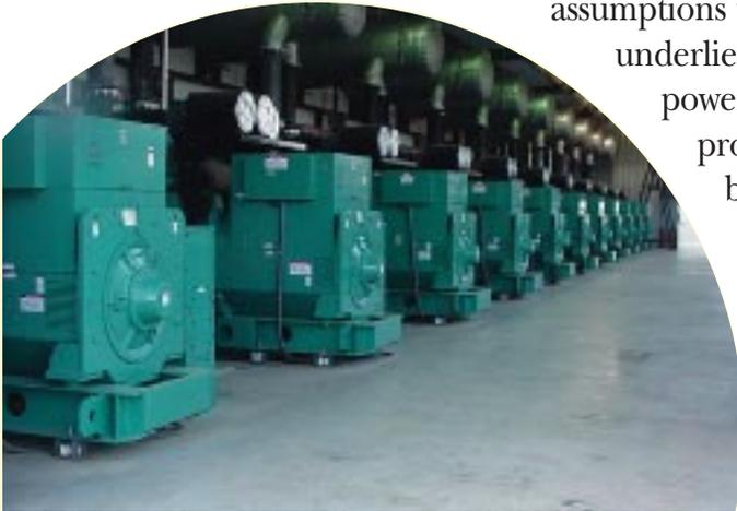
McMinville (Tenn.) Electric System installed 11 two-megawatt diesel generators to meet peaking needs in the Tennessee Valley.
